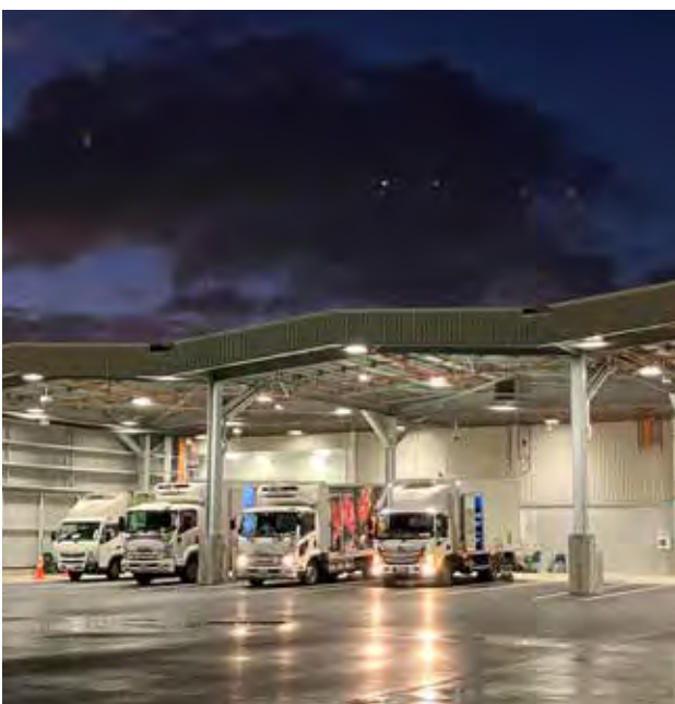
The new truck dock at the western end of the international terminal.
