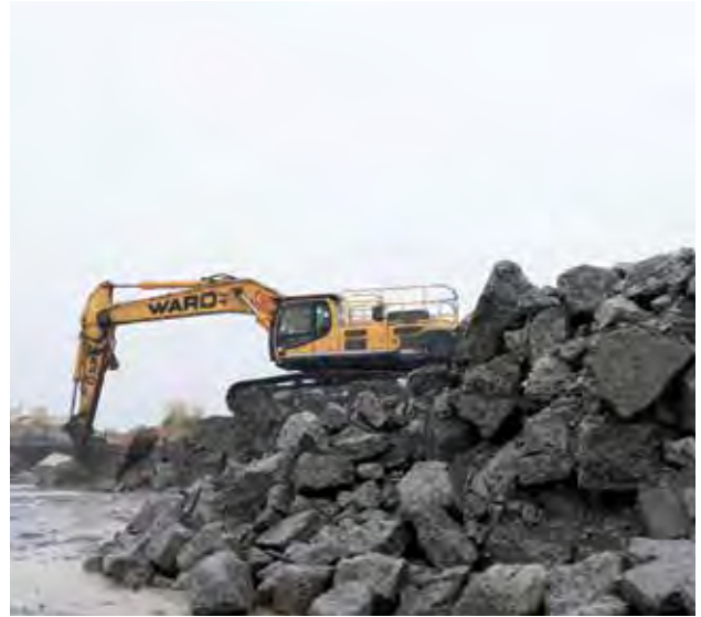
Waste concrete being recycled for the northern airfield project
